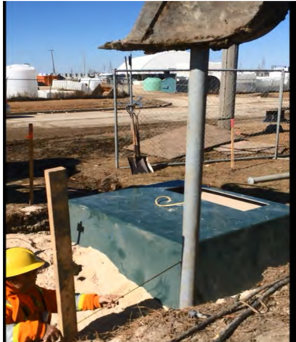
Backfill and Install Bollards
